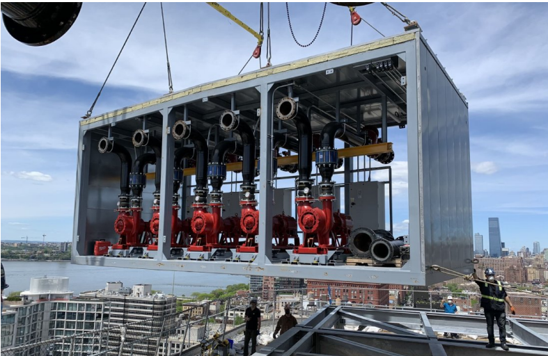
Modular HVAC equipment for an office building (credit EJS New York).
