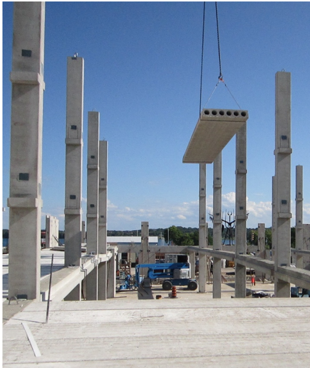
Maple Avenue Tower, a 17-storey Condo (with a 4-storey precast concrete parking garage and composite transfer slabs at the 5th floor) and Mixed Retail (Total Precast Concrete Building) in Barrie, Ontario (credit: Stubbe's Precast).
