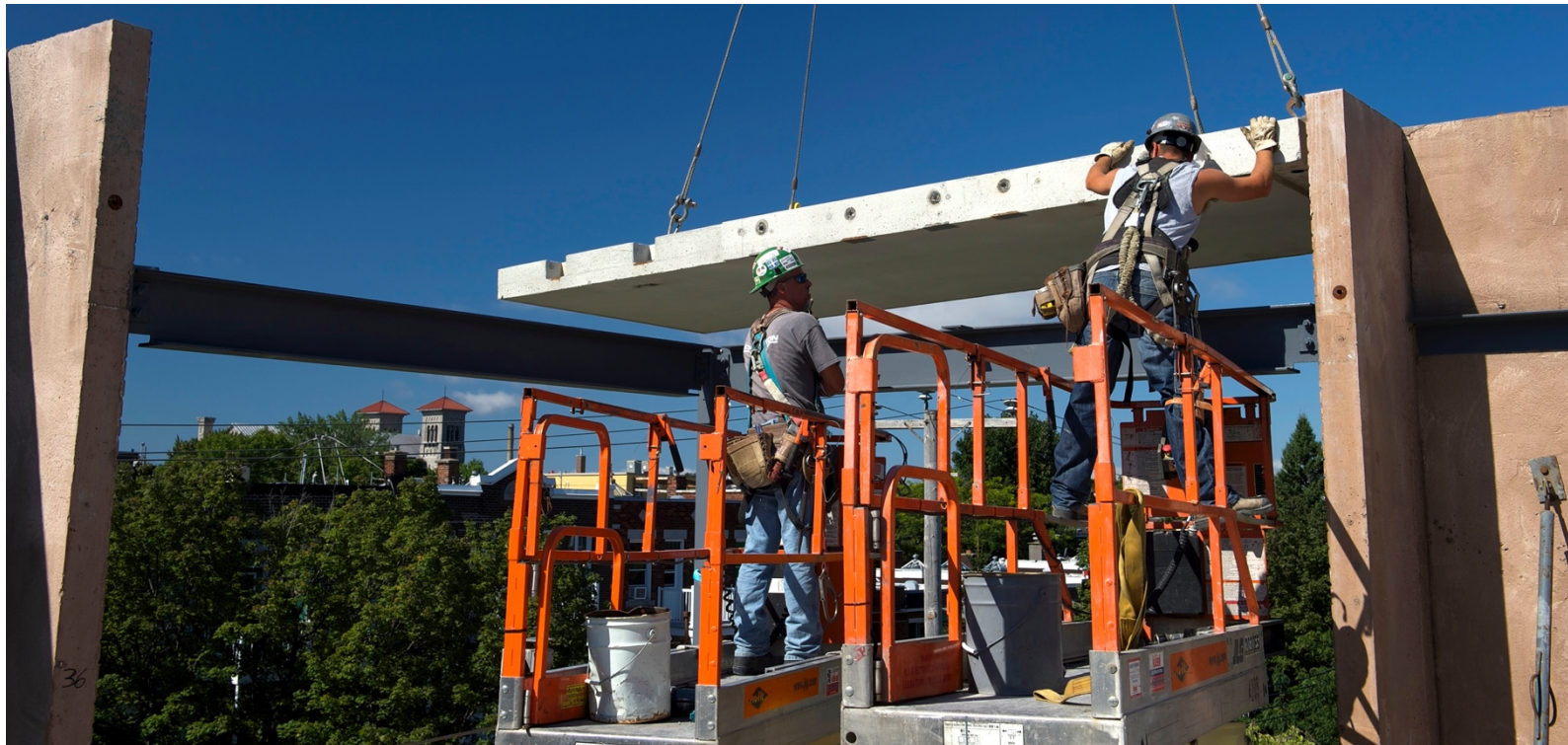
buildings in Montreal, Quebec (credit: Schokbeton & Saramac).
