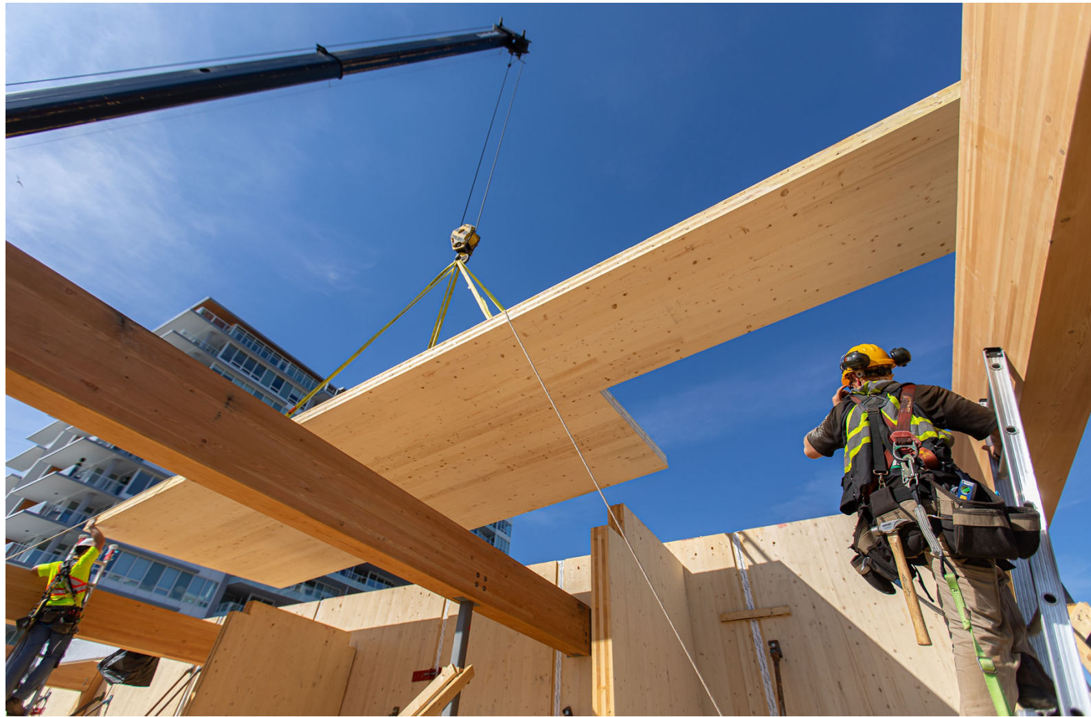
Prefab glulam and mass timber installation in North Vancouver, British Columbia (credit: Naikoon Contracting Ltd.)
