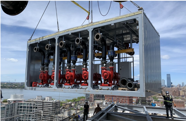
Modular HVAC equipment for an office building (credit EJS New York).
