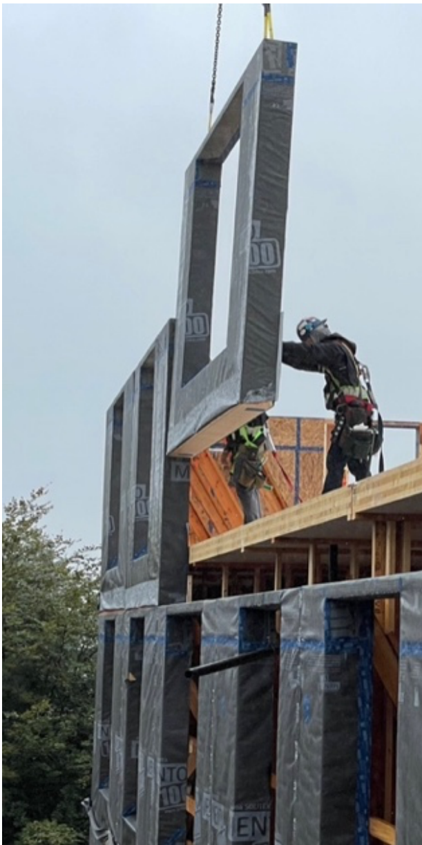
Vienna House National Housing demonstration project in Vancouver showcases the use of prefab light wood frame wall panels and mass timber floors (credit: Kelly Walsh, Sciuss).
