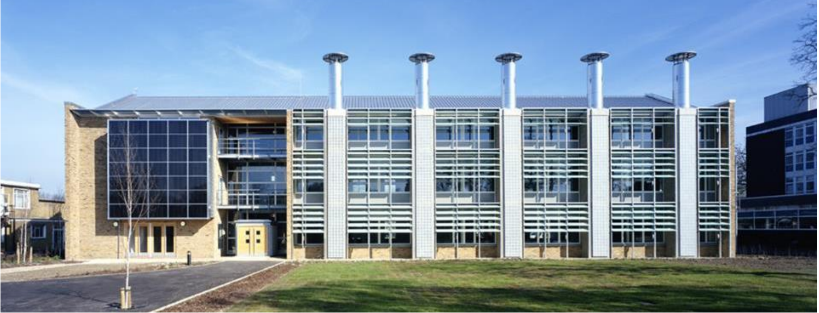
Figure 7: The BRE “Office of the Future” was designed to be deconstructed. Photo credit: BRE
