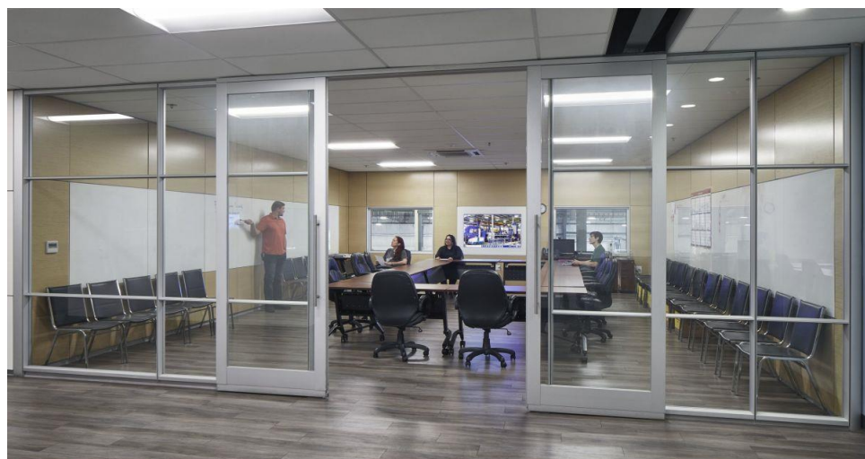
Figure 16: APEL Office renovation using DIRTT’s re-usable modular partitioning system. Image credit: DIRTT
