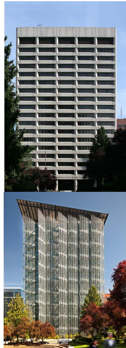
Figure 13: Edith Green Wendell Wyatt (EGWW) Federal Building before (top) and after (bottom) a whole building renovation and energy retrofit. Photo credit: Sera Design
