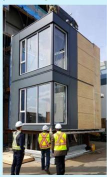
**Full-scale mock-ups** were constructed of various sections of the building to validate decisions such as connection details with column and slab, connection with the slab and concrete core and confirm the choice of steel assembly for the structural columns (Figure 28 and Figure 31).
