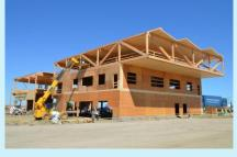
Figure 10 - Pre-fabricated elements such as large trusses were installed in the Mosaic Centre (image © Western Archrib, sourced from Wood *WORKS*! case study and Fast & Epp)
